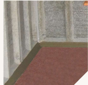
Sand and cement fillet applied to interior base of panels
