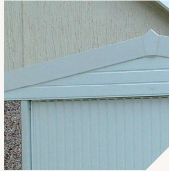
White PVCu fascias and vergeboards
